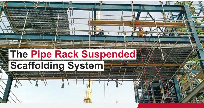
In modern industrial construction and maintenance, scaffolding serves as a crucial temporary support and working platform. The Pipe Rack Suspended Scaffolding System, as an innovative scaffolding solution, provides safe and efficient operation guarantees for complex construction scenarios and plays a significant role in industries such as petrochemical and energy.
