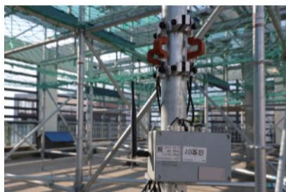
Load Monitoring System Detects the scaffolding or shoring structural load Real-time
